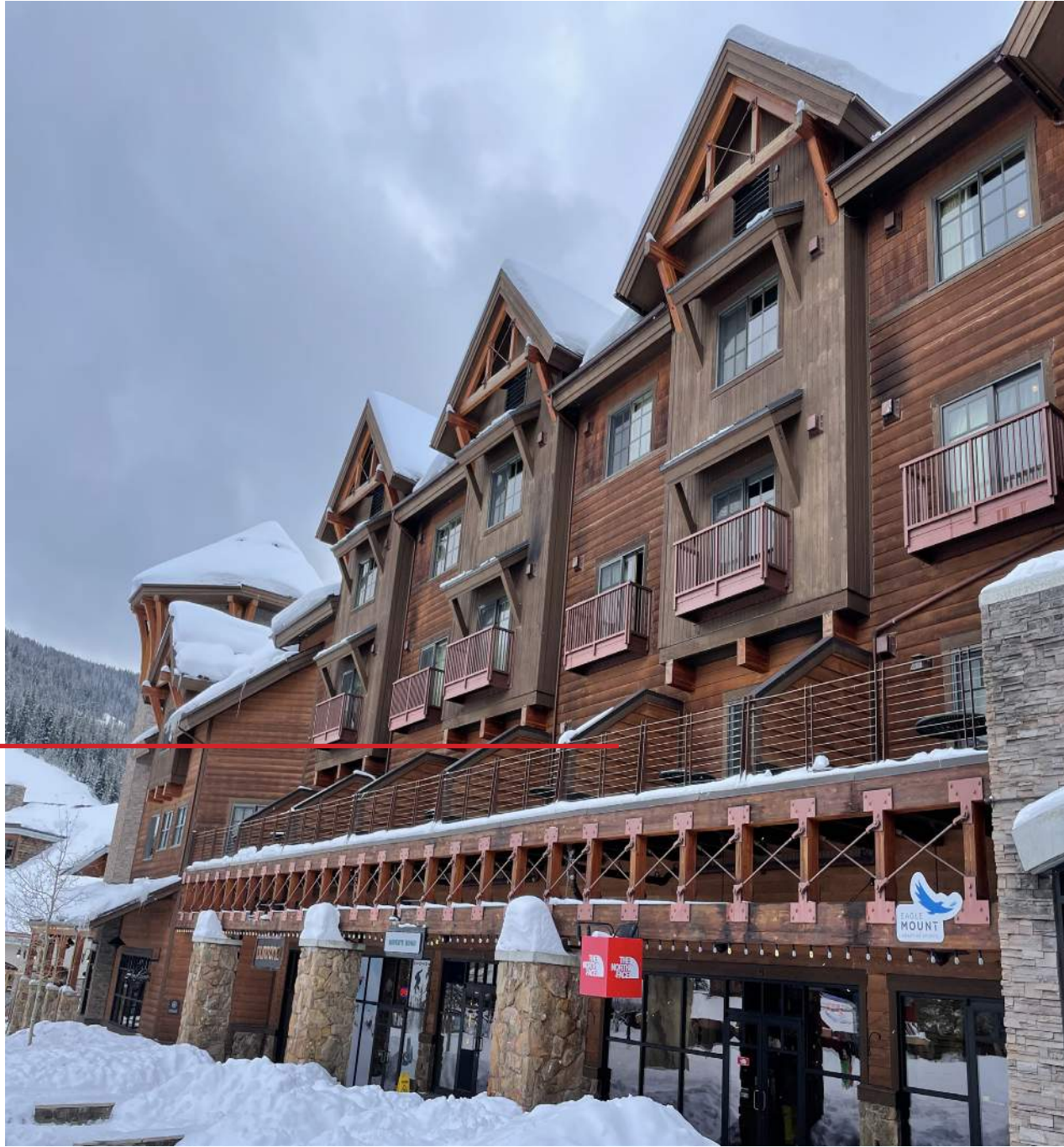
MOUNTAIN VILLAGE EXTERIOR VIEW - RESIDENCES
