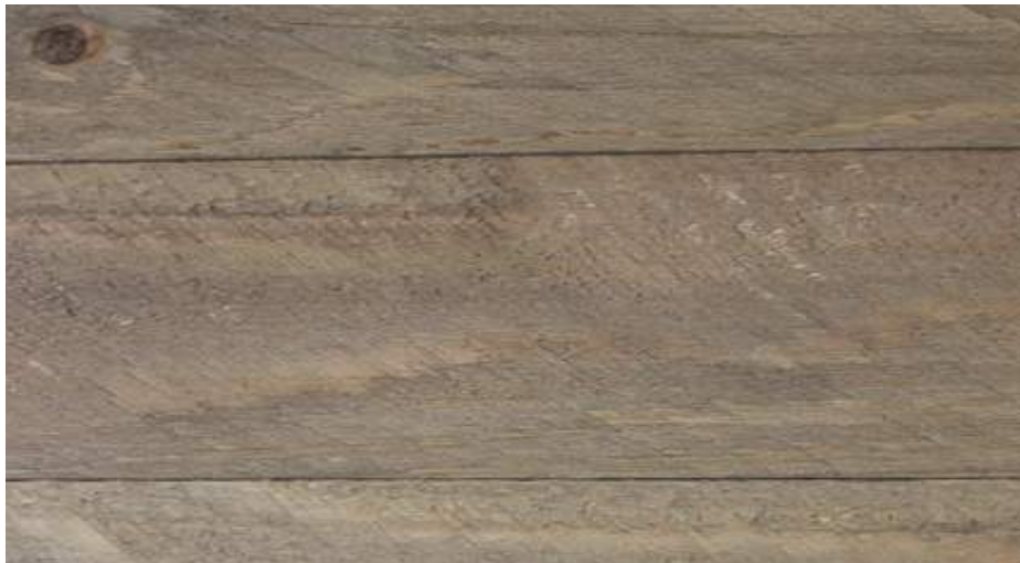
T&G SOFFIT - ELEVATOR CORRIDOR
